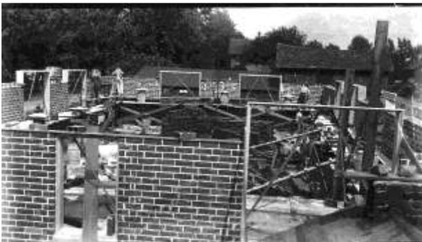
Masons are in the process of erecting the Exline building's brick walls. Notice the large stack of bricks in the center of the construction site and the wooden ramps leading to the scaffolding along the walls.
